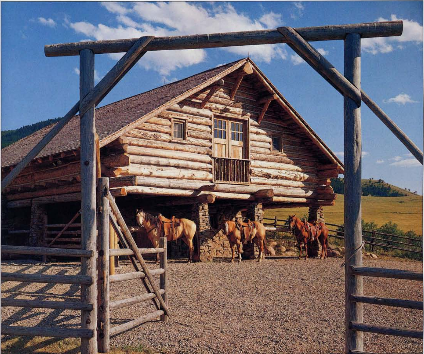
ABOVE: Saddled horses stand before the stable, which was made out of recycled pine logs and native fieldstone. "It was crafted with basic tools: a chain saw, an ax, a sledgehammer and string lines," says Howard. LEFT: A small sod-roofed fishing cabin overlooks the creek.
